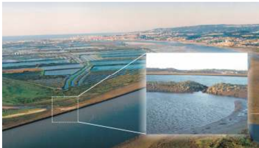
Figure 7: Detail of the communication between the two arms of the estuary at the upstream area in 1994.
